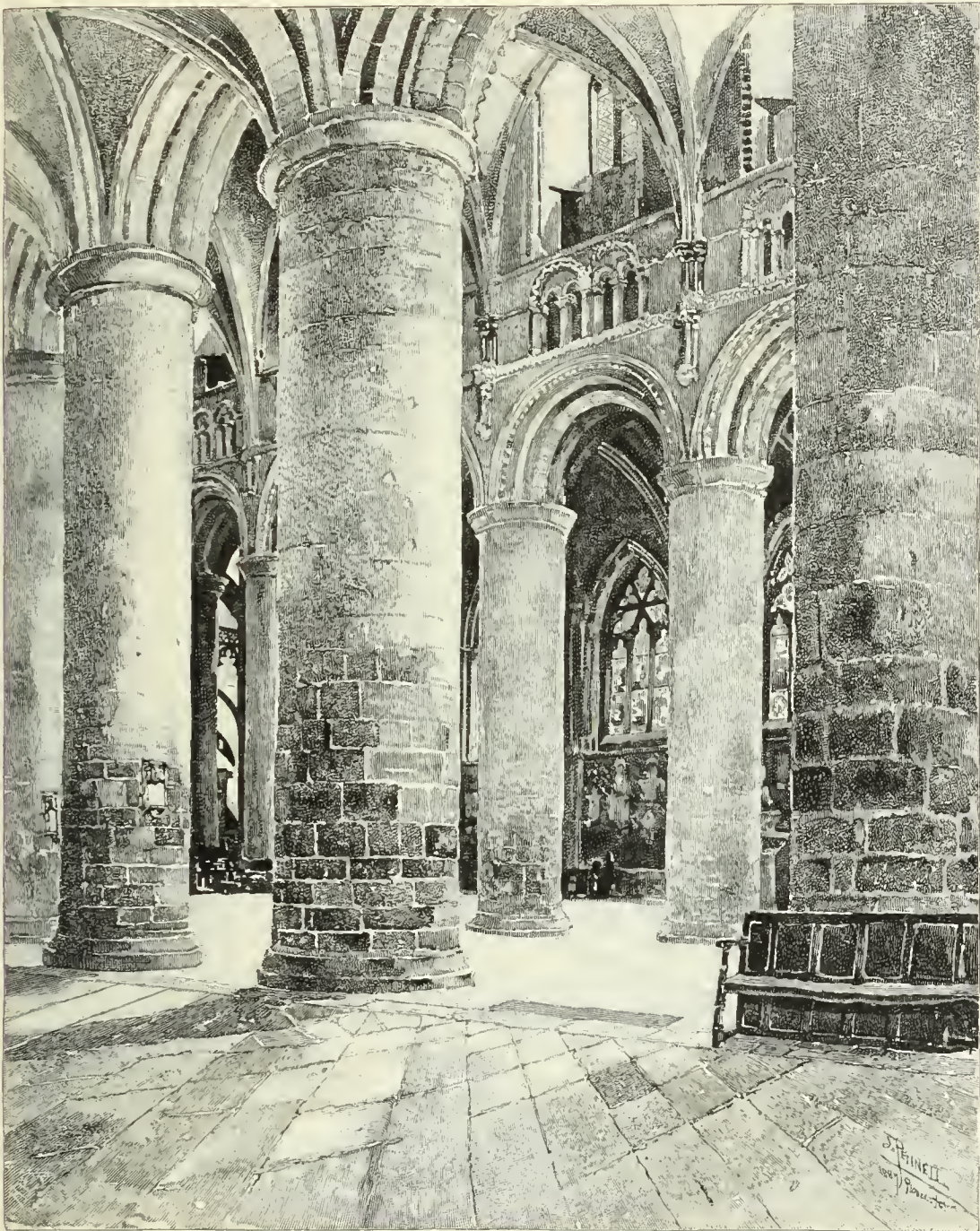
THE NAVE, FROM THE NORTH AISLE.
